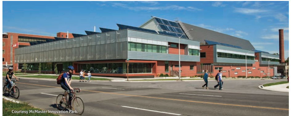
The CanmetMATERIALS building is home to 208 solar thermal collection panels and 12,000 sq ft of solar wall that are part of the MIP district heating system.
