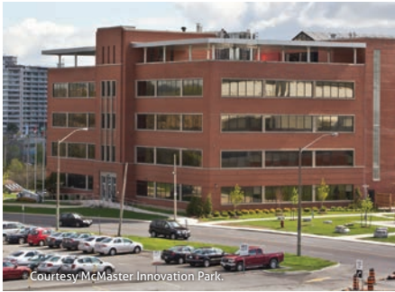
The Atrium@MIP, formerly an office and factory for Westinghouse, houses the district energy system boilers, chillers and heat pumps in a basement plant.
